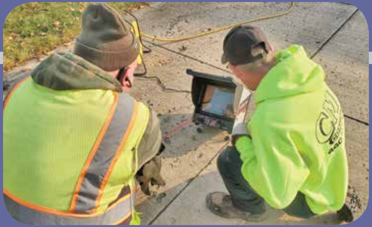
Greg Peters and Jim McCutcheon huddle around a monitor as they assess a sewer
