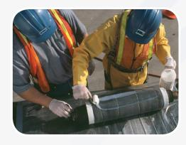
CUES-Lock Structural & Sealer Sleeves restore damaged areas to full structural strength and seals infiltration.
