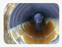
CUES-Lock Stents provides a guick and easy way to bridge holes, voids, cracks and weakened/broken sections in pipes to help and allow easy installation of any type of cured-inplace pipes through the stents. It also can be used to push sagging or delaminating cured-inplace pipes back into place.
