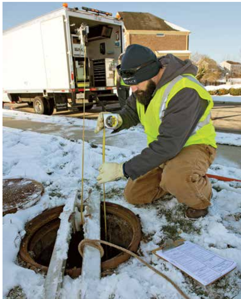
Florence Public Service Department maintenance worker Mark Teremi takes a depth measurement of a storm sewer.
