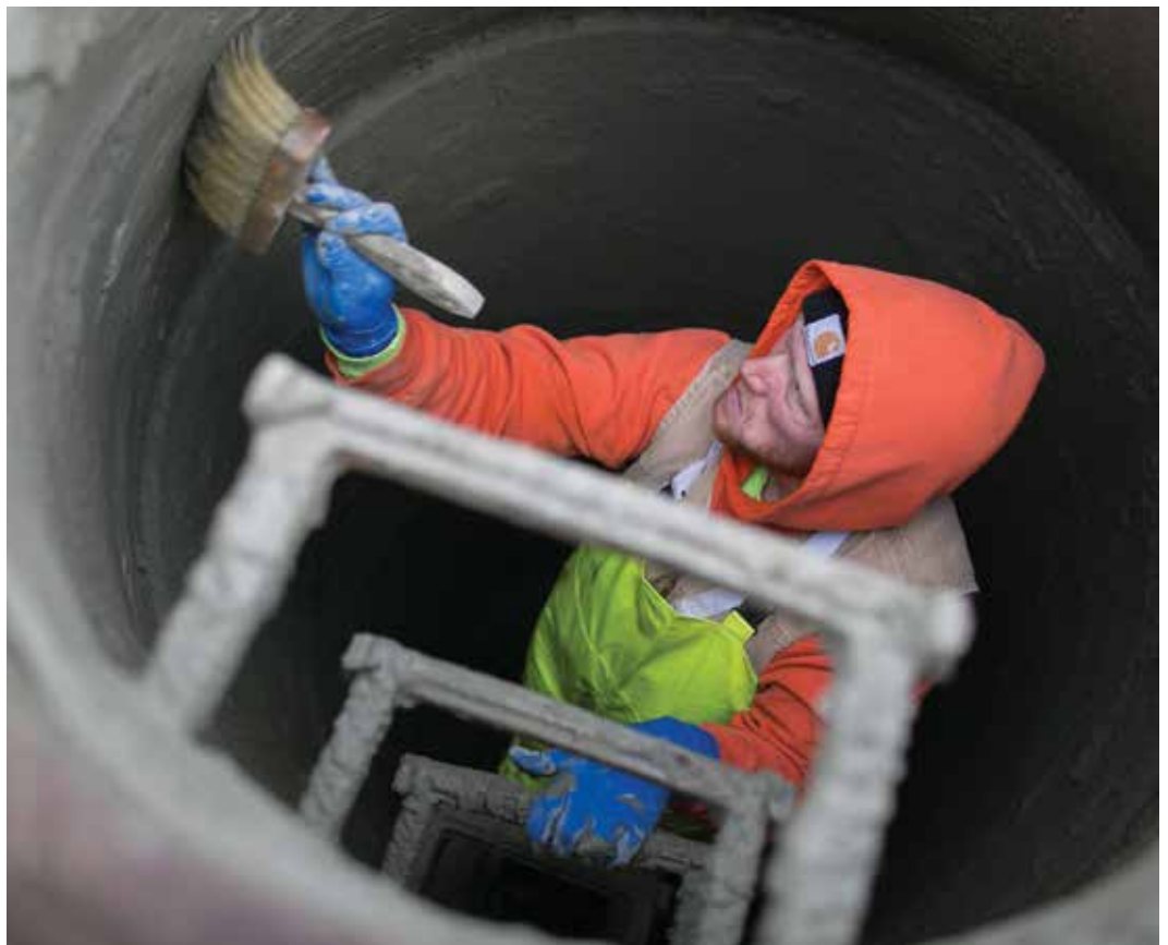
ABOVE: Cody Faucher removes a storm drain grate prior to cleaning the roadside line. >> RIGHT: Alex Faucher smoothes fresh grout inside a manhole in Lockport, New York.
