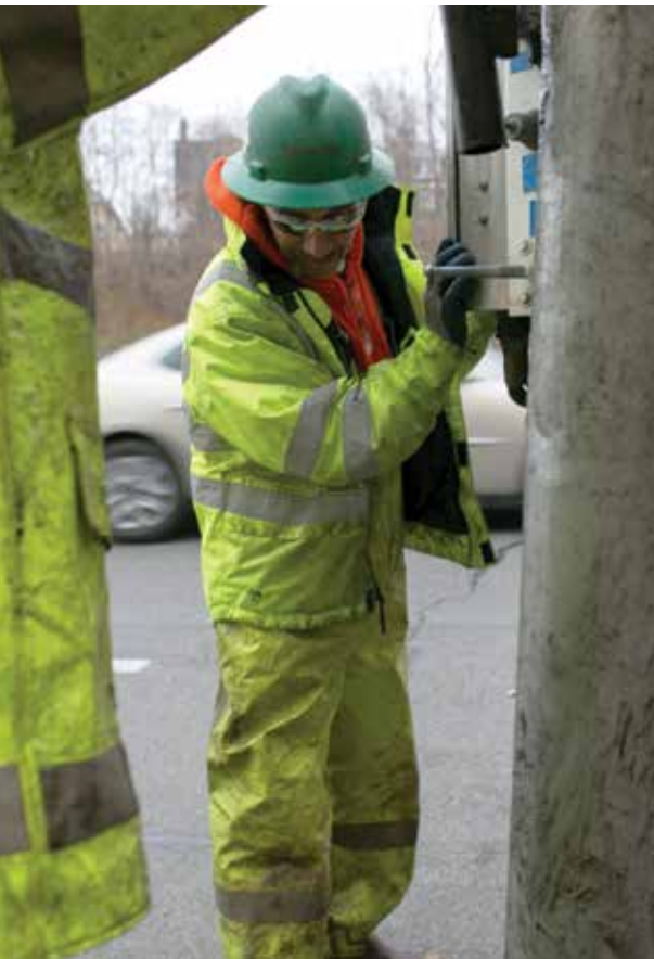
Mike Beck operates the controls of an Aquatech jet/vac truck while cleaning a stormwater line.
