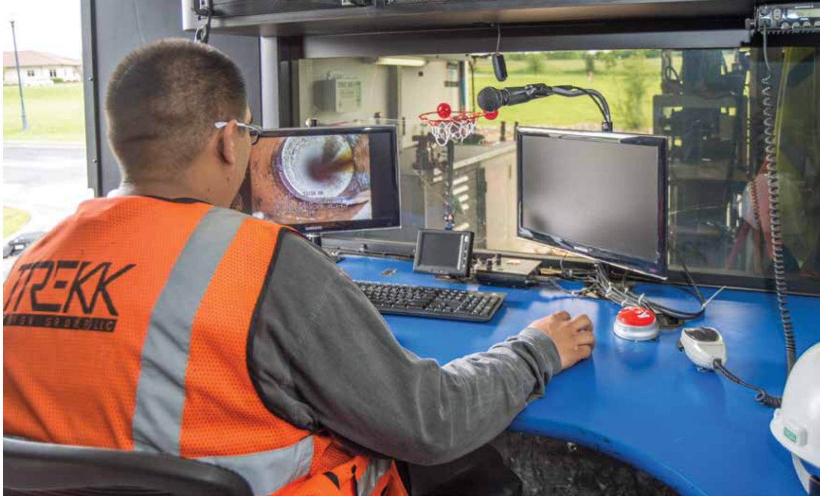
ABOVE: TREKK technician Gabe Gonzalez runs a sewer inspection from the control room of a CUES inspection van. BELOW: Gonzalez uses a winch to get the CUES Mud Master camera out of the CCTV van at the start of an inspection job.
