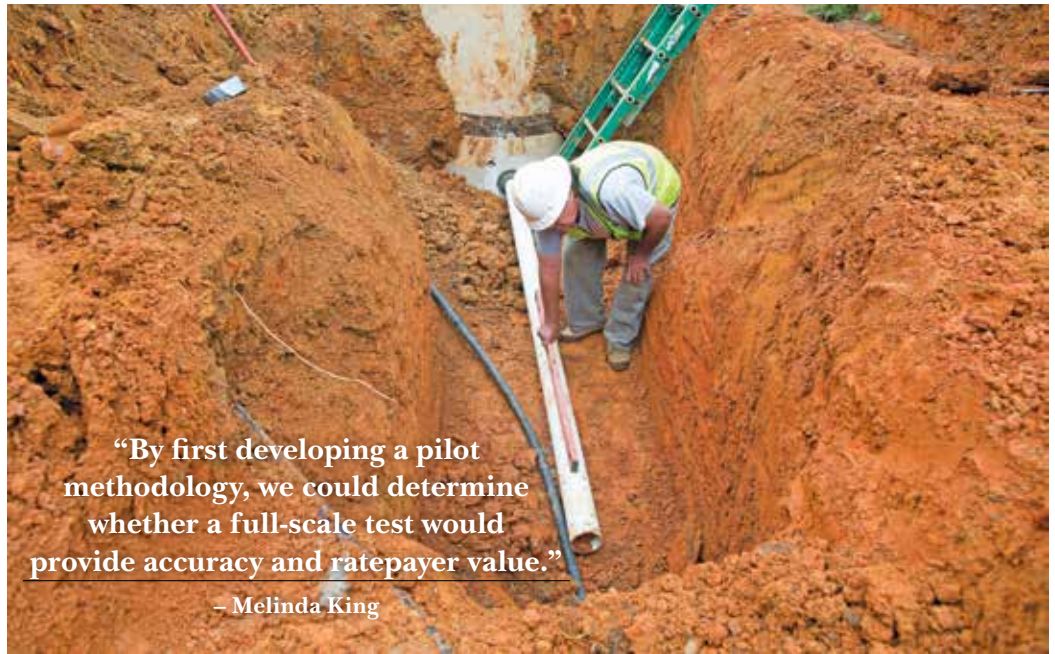
Left: Melinda King, project manager for the City of Greensboro Water Resources' Lynwood Lakes project, on site in Greensboro, North Carolina. The $9.8 million project includes 26,000 feet of water line and 30,000 feet of sanitary sewer line to serve 300 residences. Right: Workman Ed Davis uses a level to make sure a new section of pipe is set at the proper grade.
