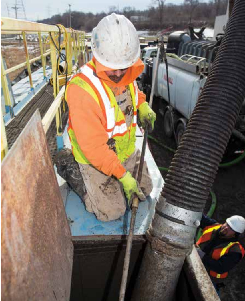
Jamey Severn uses a pressure washer connected to a Vacall hydroexcavator to loosen sediment from a dewatering tank.
