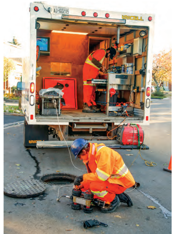
LEFT: An inspection crew lowers a camera into a remote manhole to inspect the line. Proper setup and technique is important on every job. BELOW: Equipment care and maintenance are critical parts of training. The success of an inspection program is based on the ability to maximize efficiency in the field.
