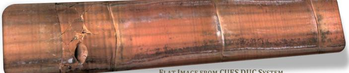
**FLAT IMAGE FROM CUES DUC SYSTEM** 8" VCP with Multiple Cracks Around Lateral Connection
