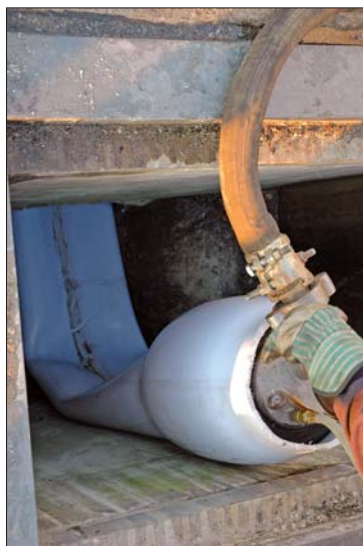
Above, the liner is heated with steam to prepare it for installation. Below left, the liner is pulled into a storm drain.
