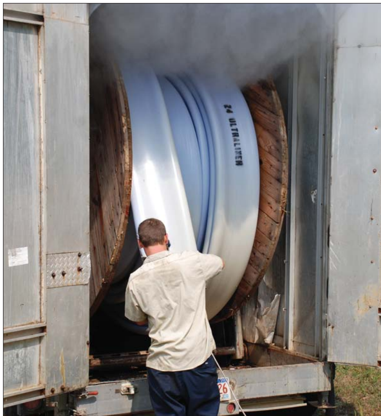
Above, the liner is heated with steam to prepare it for installation. Below left, the liner is pulled into a storm drain.
