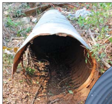
This culvert beneath a road had deteriorated badly.
