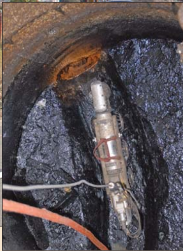
A camera from CUES Inc. is used to document sewer lines that have been cleaned.
